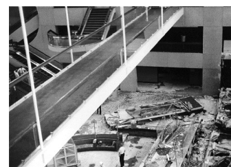
On July 17, 1981, a walkway collapsed at the Hyatt Crown Center Hotel, two months before ASTR was scheduled to meet at the Kansas City convention facility.
